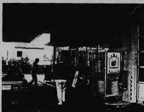
Cylinder service station
